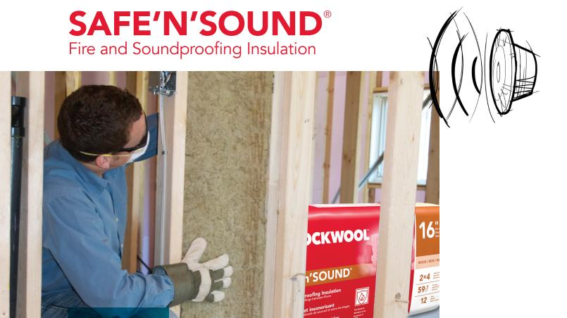
ROCKWOOL SAFE'n'SOUND® is a stone wool insulation for use in interior partitions of residential wood and steel stud construction where superior fire resistance and acoustical performance are required.
