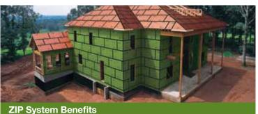
Superior Moisture ResistanceContinuous vapor permeable<br/>moisture barrier that blocks out<br/>liquid water but still allows walls<br/>to dry out.Ease of InstallationNo more delays because of felt or<br/>building wraps blowing off.Energy EfficiencyCode-recognized built-in weather<br/>and air barrier.
